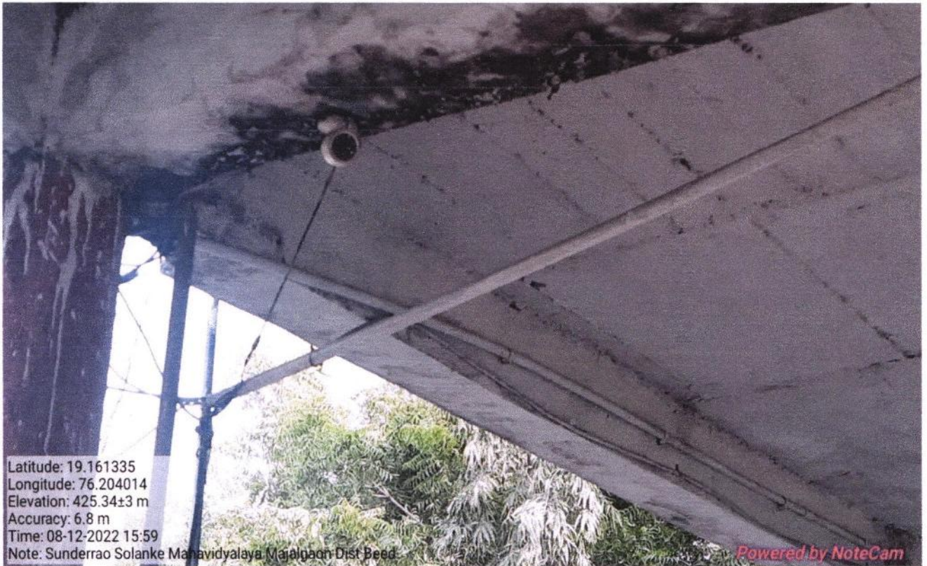
CCTV Camera at Arts Building
